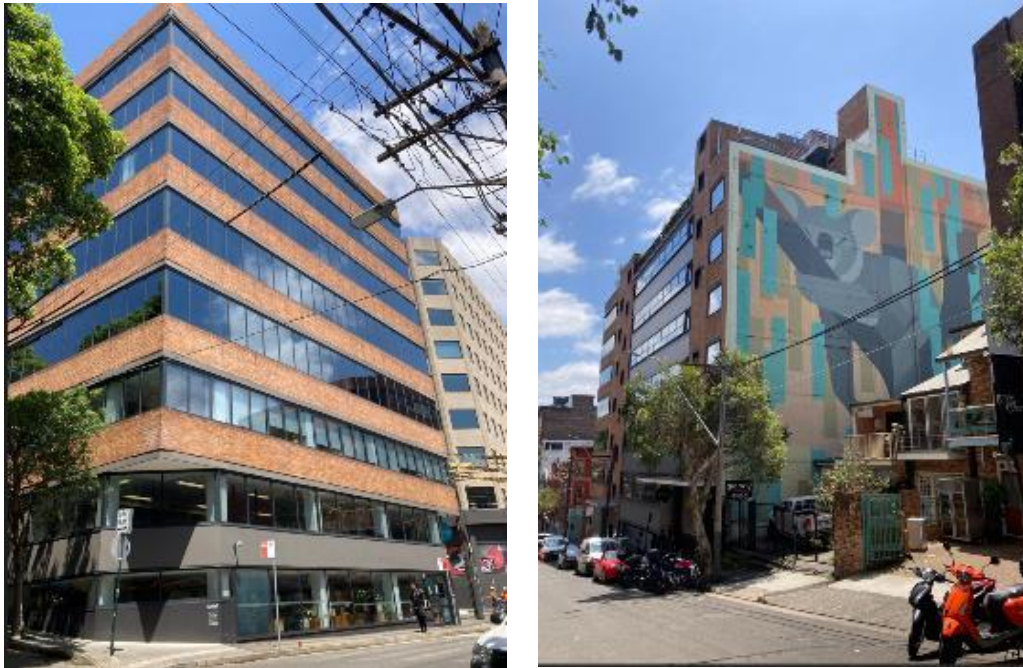
Figure 14: Canva premises at 110-120 Kippax Street to the east of the site, including public art.
