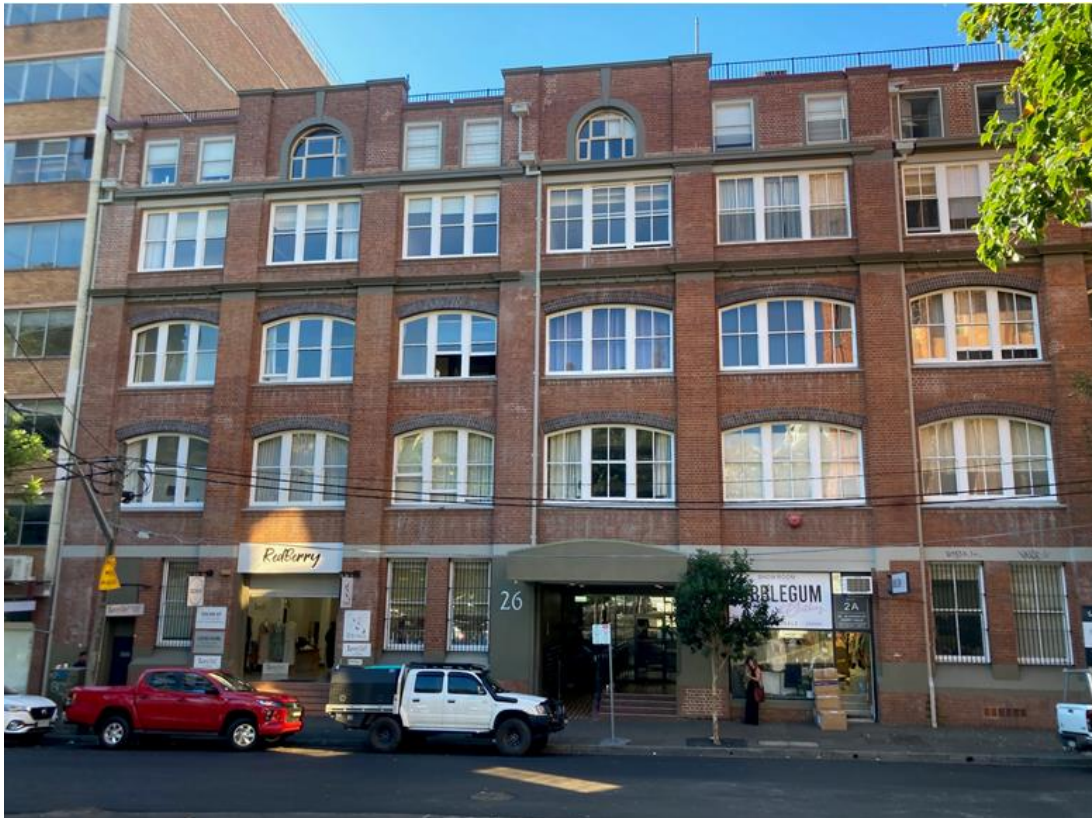
Figure 8: Mixed use building at the eastern property boundary (26-44 Kippax Street).
