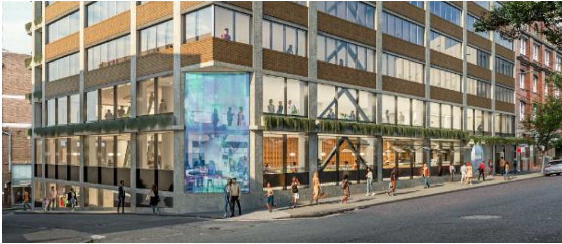
Figure 46: Extract from photomontage, showing projecting planter boxes and planted awning at the Kippax Street and Terry Street frontages.
