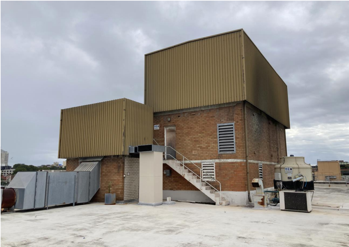
Figure 6: Plant rooms at the roof level of the site.
