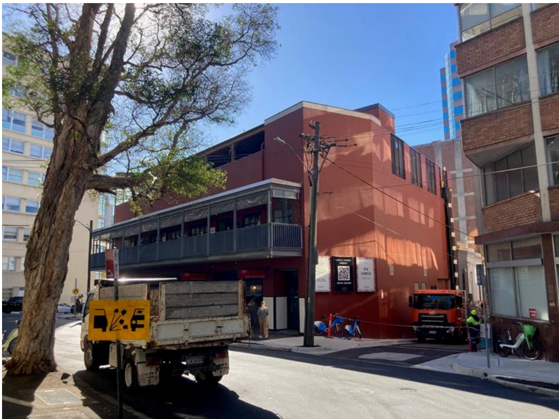
Figure 9: Aurora Hotel, west of the site (320-324 Elizabeth Street).
