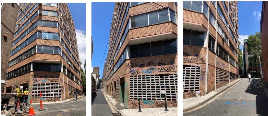
Figure 4: site viewed looking east along Sophia Street and south along Terry Street.
