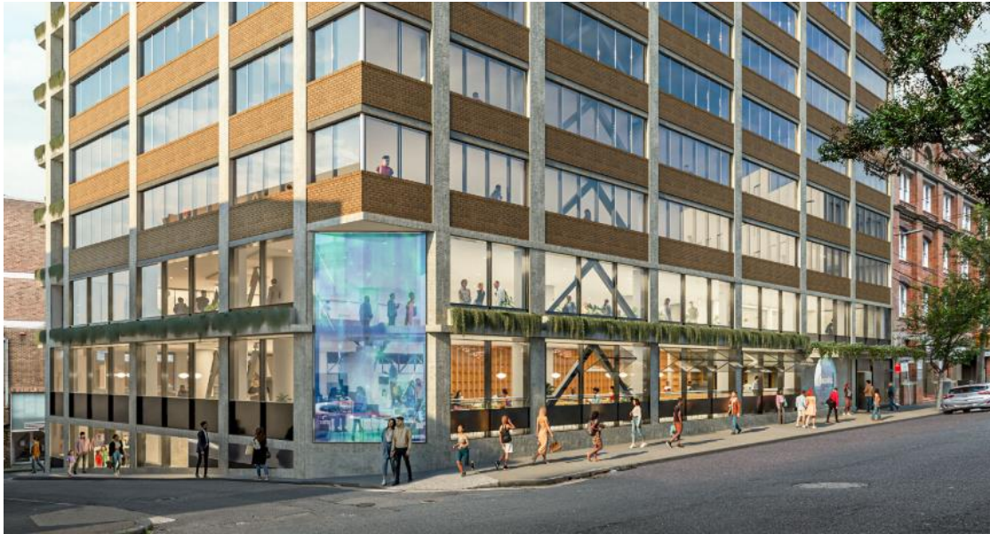
Figure 31: SIGN 2: Rectangular sign using transparent LED adhesive film applied to glazing at the corner of Kippax and Sophia Streets.
